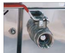
Safety lock ball valve drain
